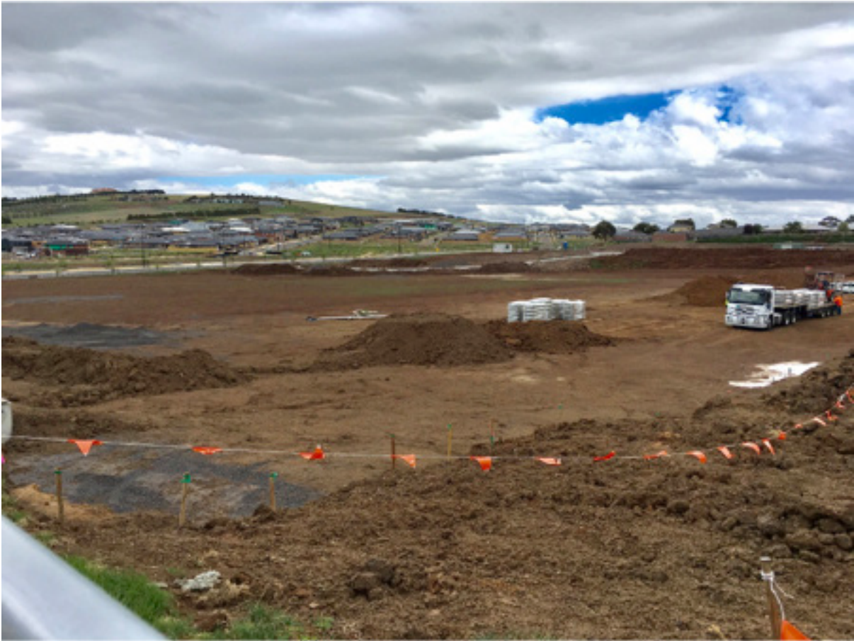
IMAGE 4 - Construction of the Woolworths site
