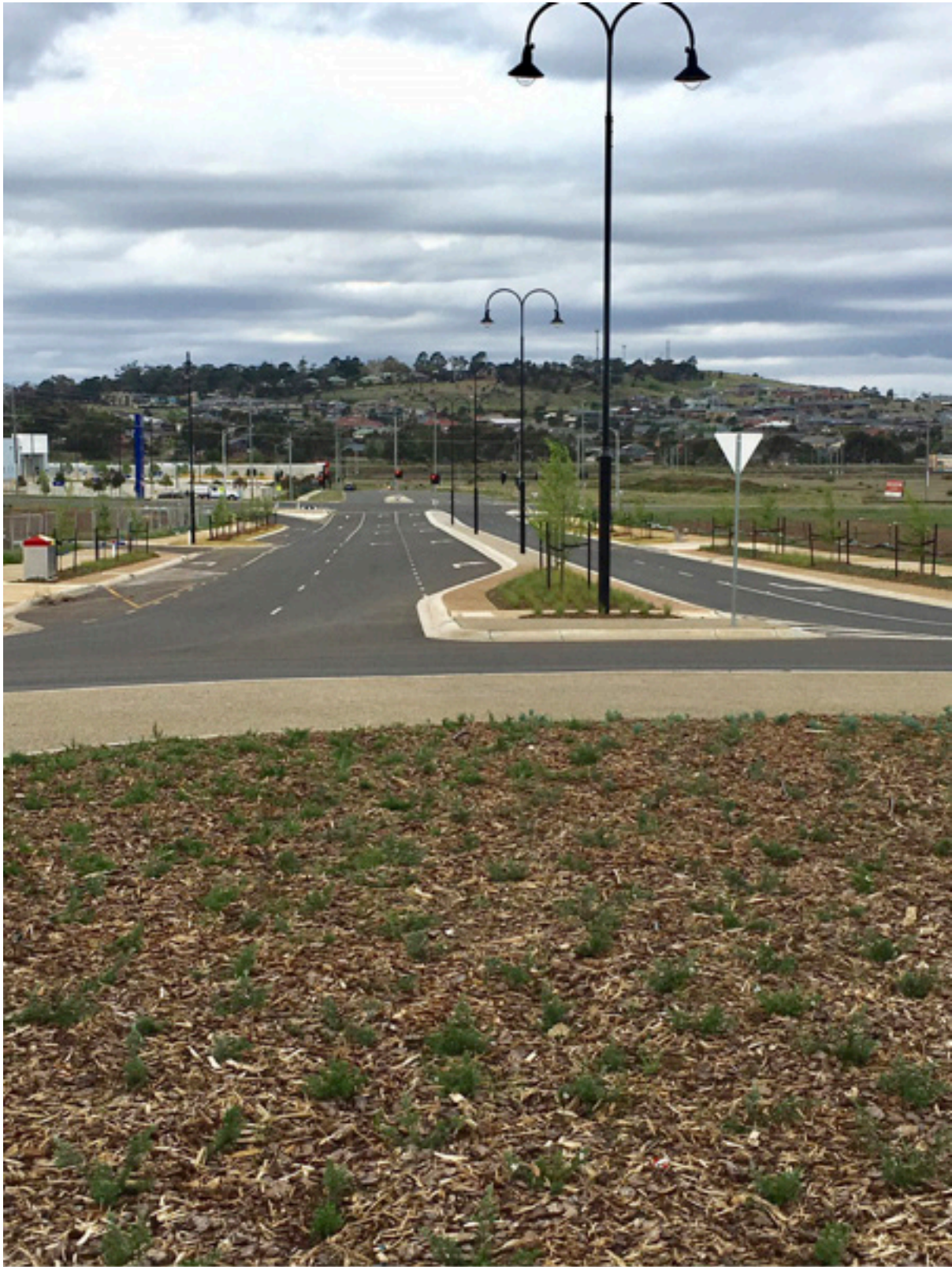
IMAGE 2 - Completed & landscaped roundabout at the corner of Elizabeth Drive & Budhurst Drive (looking east)
